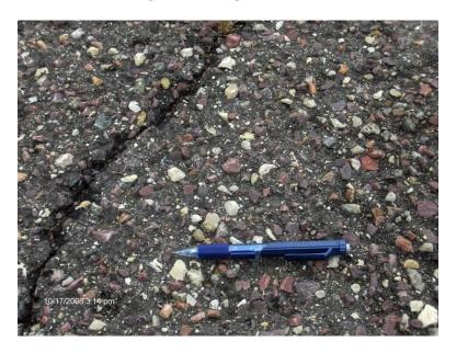
Raveling and weathering are the wearing away of the pavement surface. Raveling is the condition where the mid- to large size aggregates are becoming dislodged; weathering is when the fine aggregate wears away exposing the edges of the larger aggregate. These distresses are usually evident over large areas and may occur together (pictured above) or separately. Raveling and weathering may indicate that the asphalt binder has hardened significantly.
